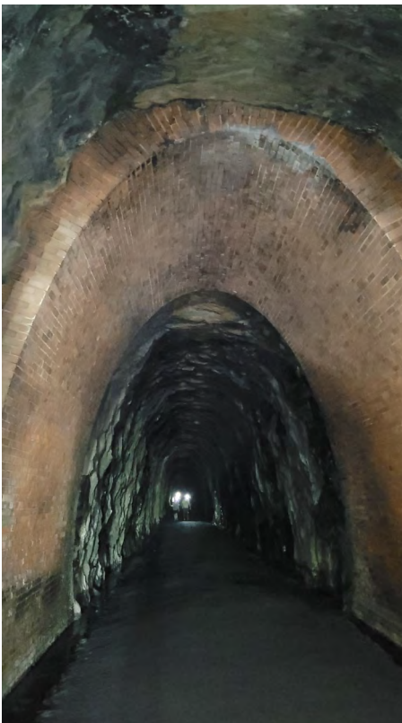
The Crozet Tunnel from the inside. Photo by Ben Johnson
